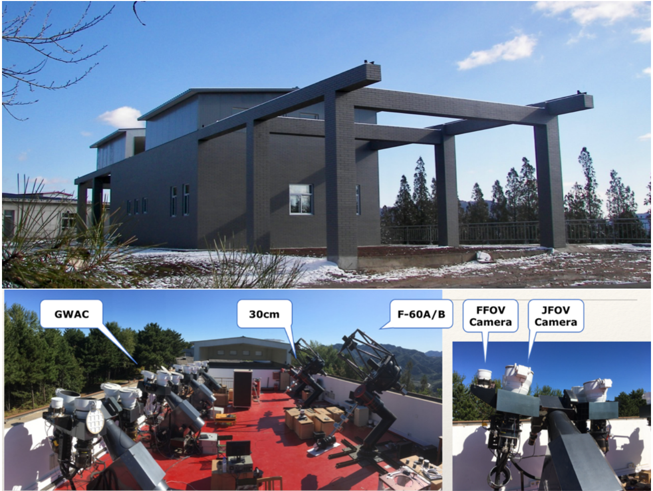
Figure 1. Top: The dome of the GWAC. The roof can be opened along the rails. Bottom left: the telescopes of the GWAC-A, the GWAC-F60A/B and the GWAC-F30. Bottom right: two types of cameras (JFoV and FFoV camera) mounted on one GWAC mount.
